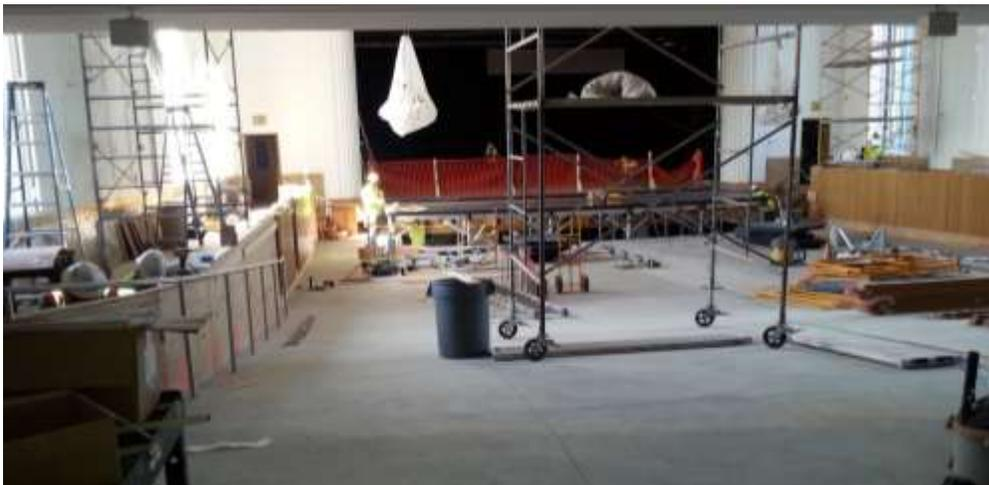
You can see the new shutters, which can cover the windows or be left open for sunlight, They are composed of acoustic materials, a change, one of several, which should improve the hall's sound. On the left and right, you can see where the new parterres are going. There will be no center aisle. Patrons will use aisles alongside the parterres. If you are seated in the parterre area, you will be on the same floor level as the stage. What a view!
